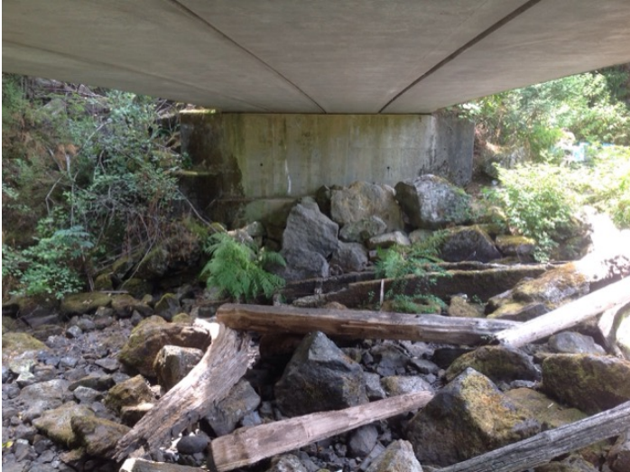
Right Bank Abutment when facing downstream
