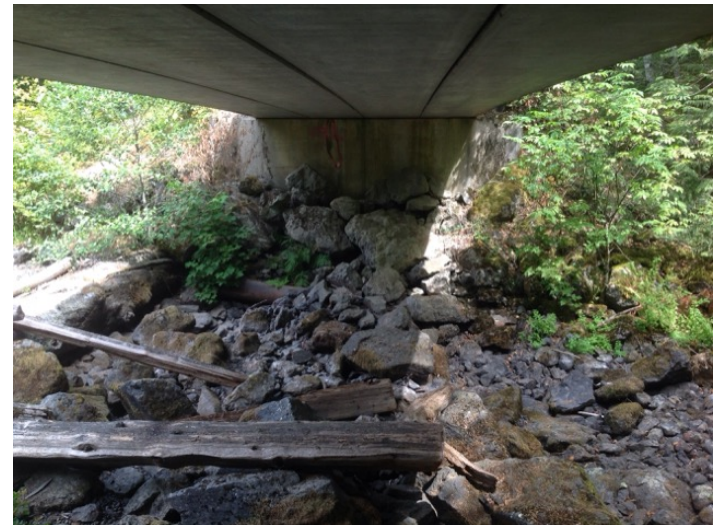
Left Bank Abutment when facing downstream
